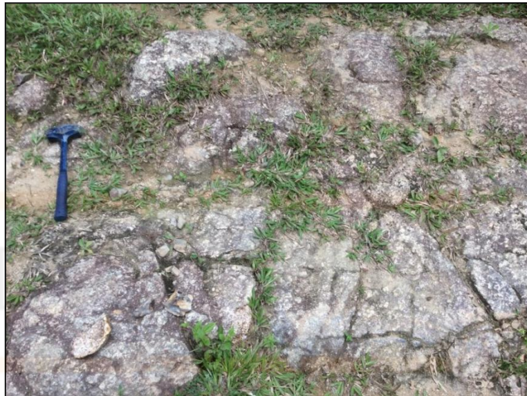
Figure 4.18: Physical weathering that undergo by granite outcrop
