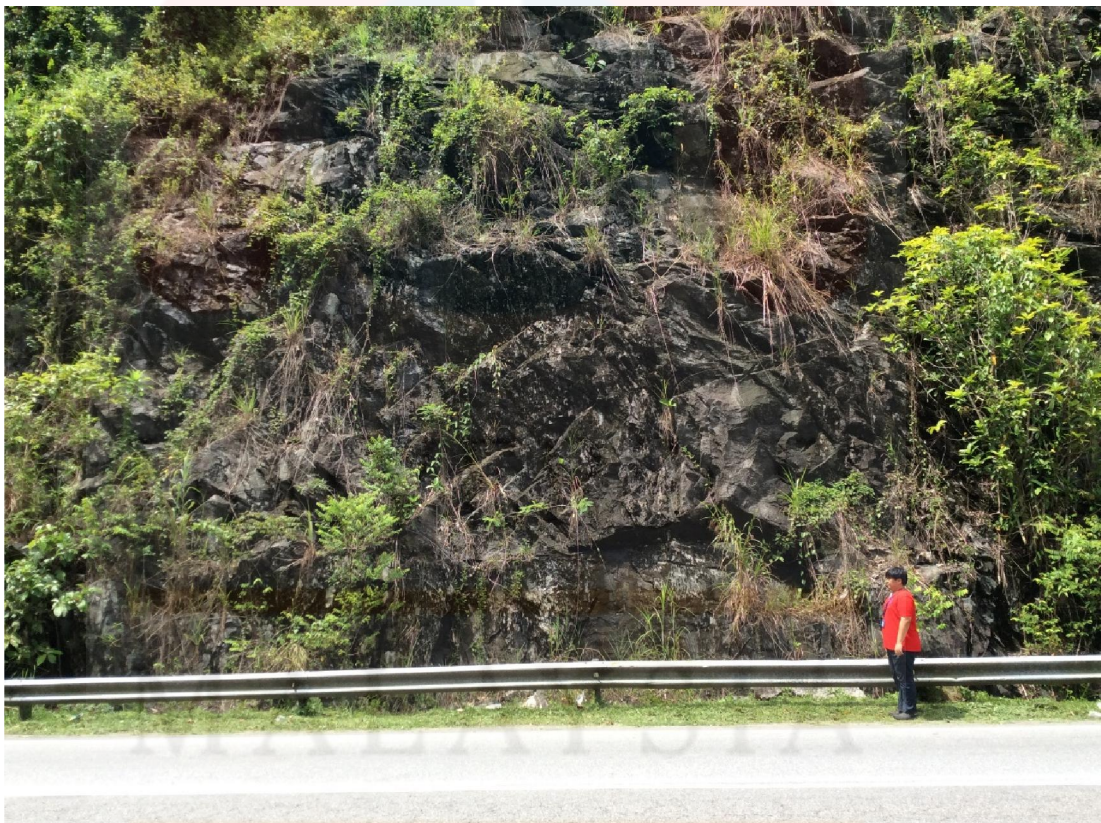
Figure 5.1.2: Photo taken at Slope 1
