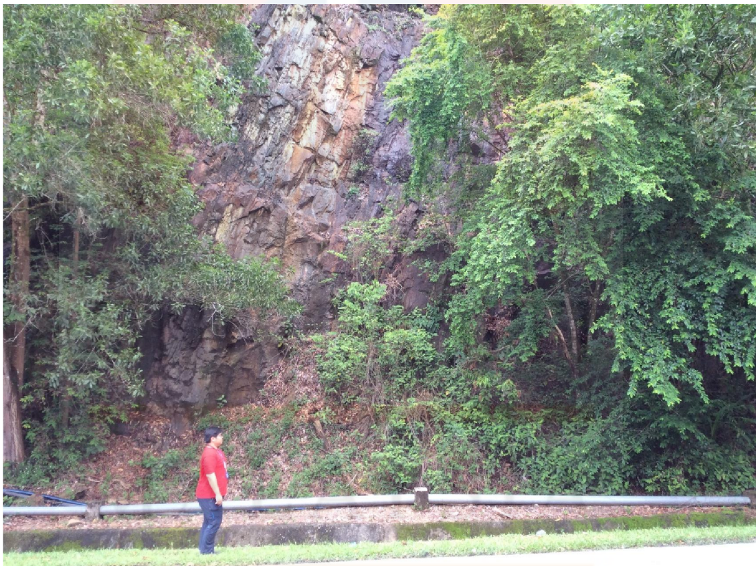
Figure 5.1.5: Photo taken at Slope 3B
