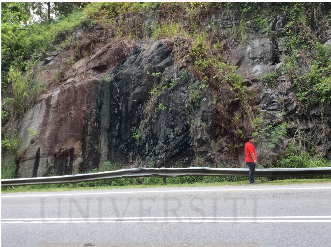
Figure 5.1.3: Photo taken at Slope 2
