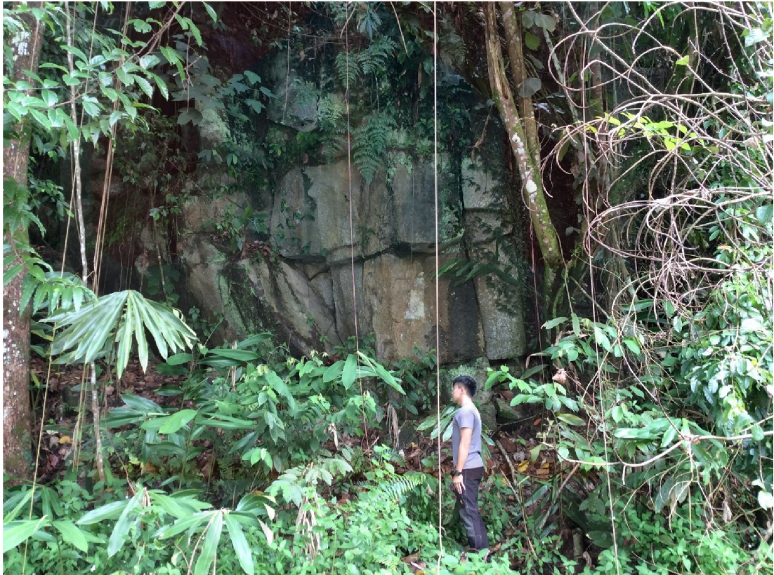
Figure 5.1.6: Photo taken at Slope 4
