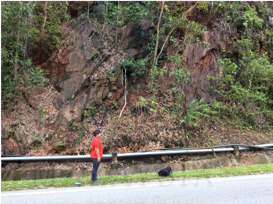
Figure 5.1.4: Photo taken at Slope 3A
