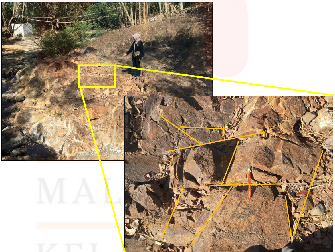
Figure 4.44 : The non systematic joint at alteration of lava at the Pentung River.
