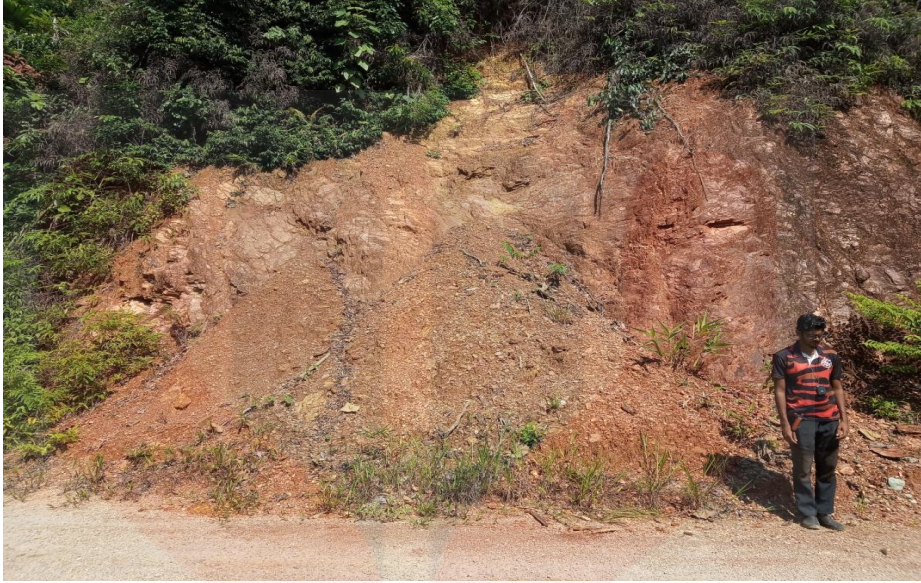
Figure 4.3: Example of mass wasting in study area
