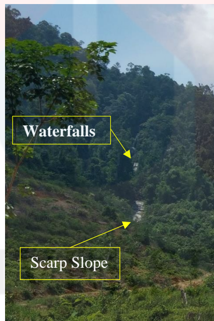
Figure 4.4: The waterfalls with scarp slope showed.
