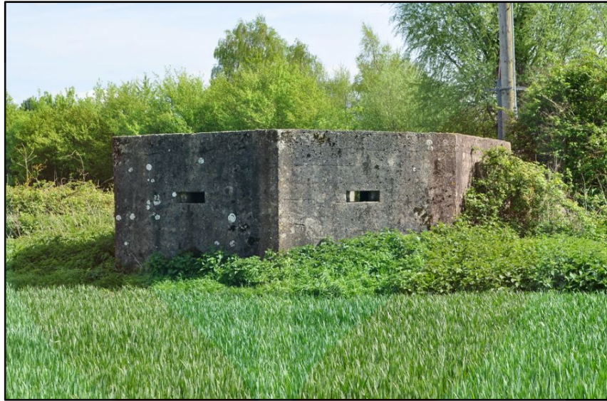
GAMBAR 2.7 : Kubu kebal tipologi Type 24 (FW3/24) yang terdapat di GHQ Line (General Headquarters Line), Moor Park, Farnham GU10, United Kingdom
