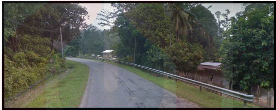
Figure 4.2: Road at KM34 Jalan Jeli-Dabong near the Kuala Balah.
