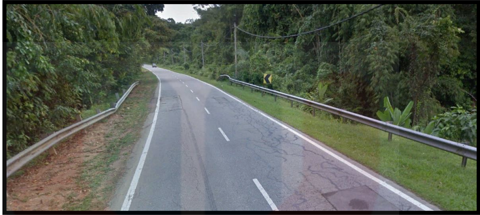
Figure 4.1: Road at KM37 Jalan Jeli-Dabong near Kg Reka.
