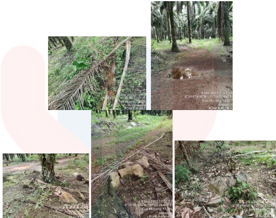
Figure 5.7: Stagnant rainwater and boulders along line survey 2
