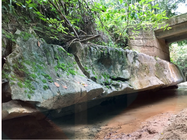
Figure 4.13 Moss grows on the surface of the limestone outcrop.
