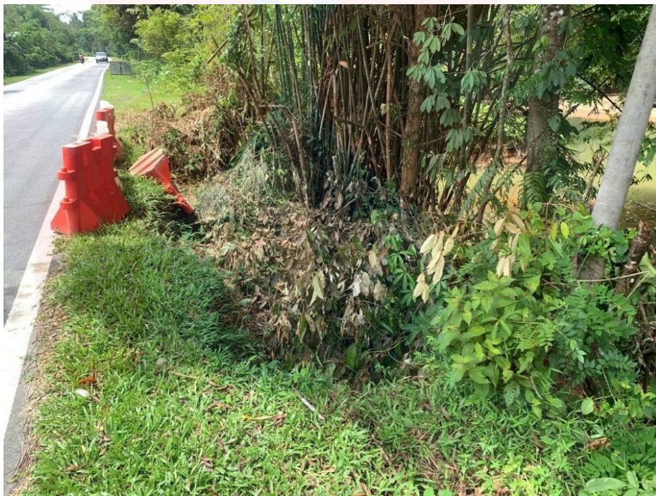
Figure 5.4: The ongoing landslide along the main road in Kampung Kalai.
