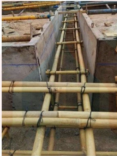
Figure 2.1.2: Bamboo as a replacement for steel reinforcement.
