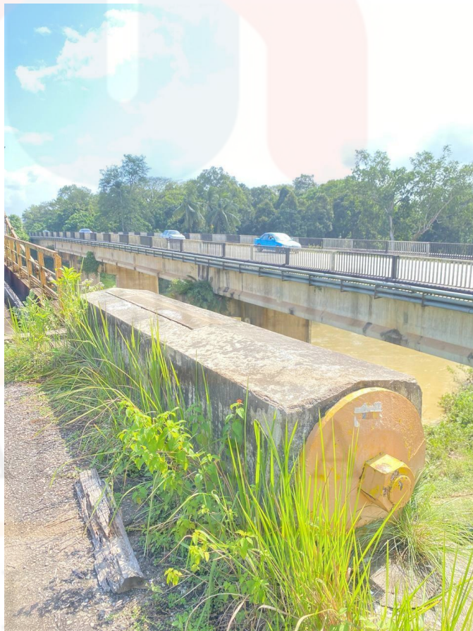
Rajah 4.17: Anchor Jambatan Gantung, Sultan Ismail, Kuala Krai, Kelantan
