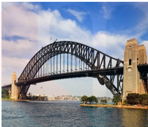
Gambar 2: Sydney Harbour Bridge, Sydney, Australia
