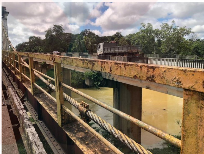
Rajah 4.8: Susur tangan (Handrill) Jambatan Gantung, Sultan Ismail, Kuala Krai, Kelantan
