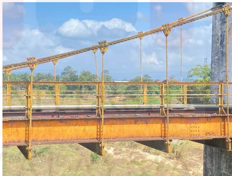
Rajah 4.16: Penyangkut (Hanger) Jambatan Gantung, Sultan Ismail, Kuala Krai,
